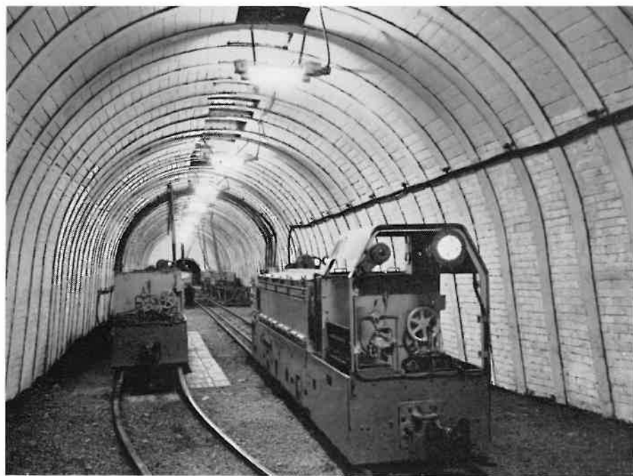
Flameproof fluorescent lighting fittings in the underground mines roadway of Heam Heath Colliery, Staffs.
