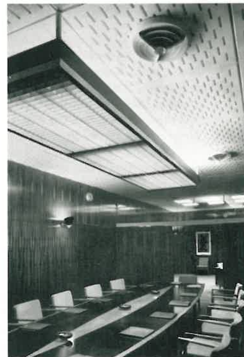
A shell concrete building illustrating the way in which difficulties encountered when providing a high level of illumination in this type of building were first solved. This is a drawing office at Swan Hunter and Wigham Richardson Ltd. at Newcastle-upon-Tyne with an illumination level of 45 lumens per square foot. The control gear for the cold cathode lamps is mounted behind the acoustic panelling. The pendant fittings contain tungsten lamps.
