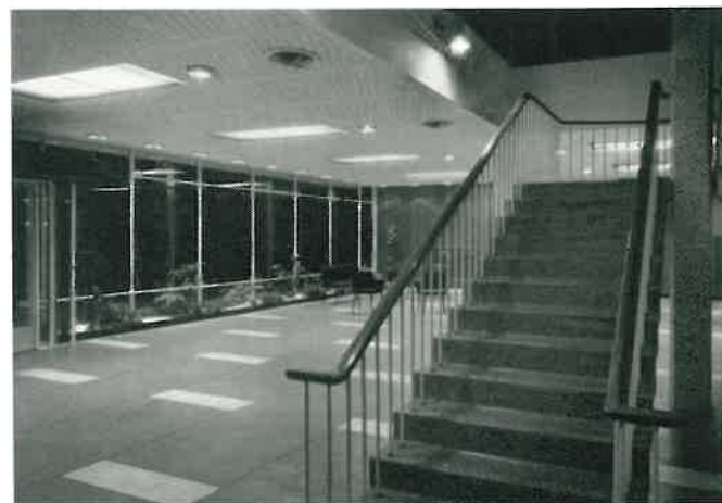
Main entrance hall of laboratory and administrative block for the Bowater Paper Corporation at Northfleet. Fibrous plaster troffers containing fluorescent lamps and control gear behind lowers act as fireproofing for the structural steel work of the building. Tungsten spotlights add sparkle.
