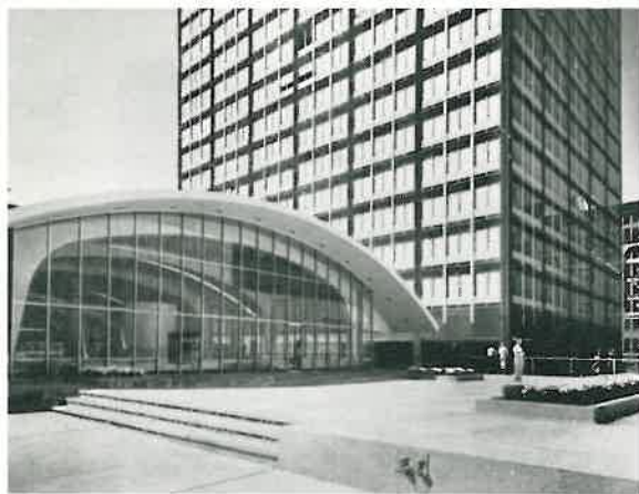
Photo—Ezra Stoller. Mile High Center, Denver, Colorado. Architects: Ioh Ming Pei. The main block of this building has large open planned offices over 70 ft. deep with a ceiling only 8½ ft. high. Here high quality artificial lighting and ventilation are necessary or the lack of direct natural lighting and ventilation will be painfully obtrusive.
