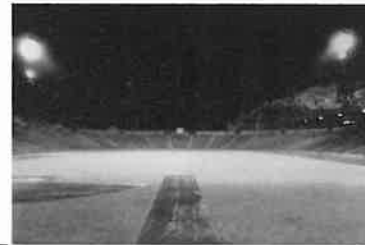
Floodlighting at the Soo Kun Poo Stadium in HongKong. Four towers with lighting grids were erected at a mean height of 174 ft. above the level of the playing field and each carried a total of 41 1500-watt A.E.I. M25 floodlights.
