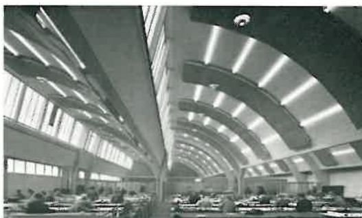
A shell concrete building illustrating the way in which difficulties encountered when providing a high level of illumination in this type of building were first solved. This is a drawing office at Swan Hunter and Wigham Richardson Ltd. at Newcastle-upon-Tyne with an illumination level of 45 lumens per square foot. The control gear for the cold cathode lamps is mounted behind the acoustic panelling. The pendant fittings contain tungsten lamps.
