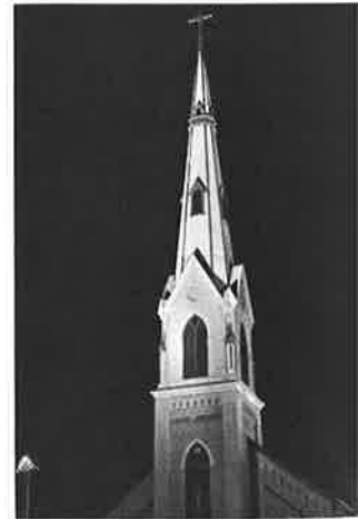
From six poles, a total of thirty 500-watt PAR-56 narrow spots are aimed at the steeple near downtown Dayton, Ohio.
