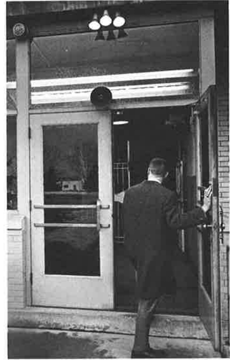
Four Power Groove lamps in two-lamp units
