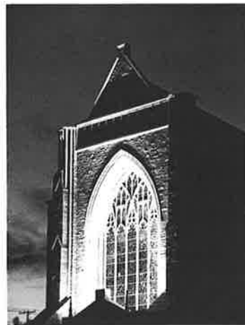
The exterior facade is lighted by 500-watt PAR-56 Quartzline lamps in units that incorporate protective cover glass.
