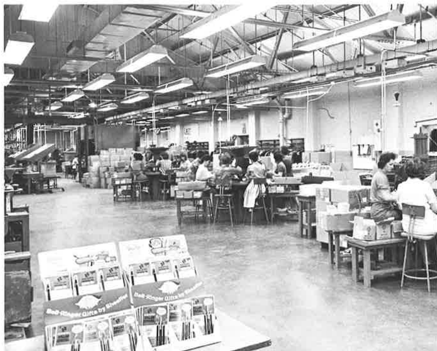
Power Groove lamps were installed in this packaging department, also. Lighting level is about 125 fc. Lamps have been in since 1962. The system is cleaned twice a year — during inventory shut-down.
