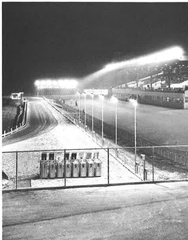
The need for a high degree of light control and good color rendition results in the use of incandescent lamps. The rectangular beam shape provided by Quartzline lamps and fixtures, and very narrow vertical beamspread and sharp cut-off characteristics are well suited to the layout of a race track.
