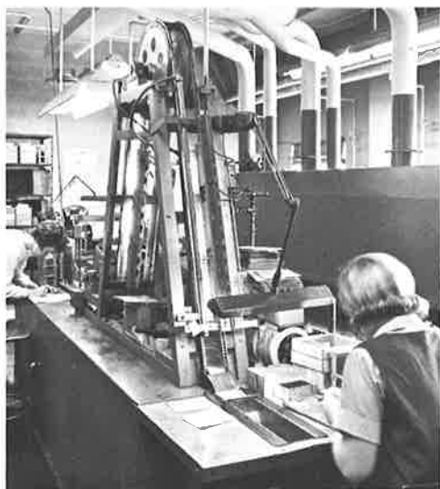
Ink cartridges are imprinted and the imprints dried quickly. Space is at a premium. By replacing PAR heat lamps with 1500-watt quartz infrared lamps time and space were reduced.
