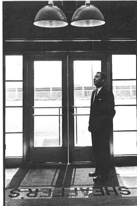
Two 400-watt color-improved mercury lamps
