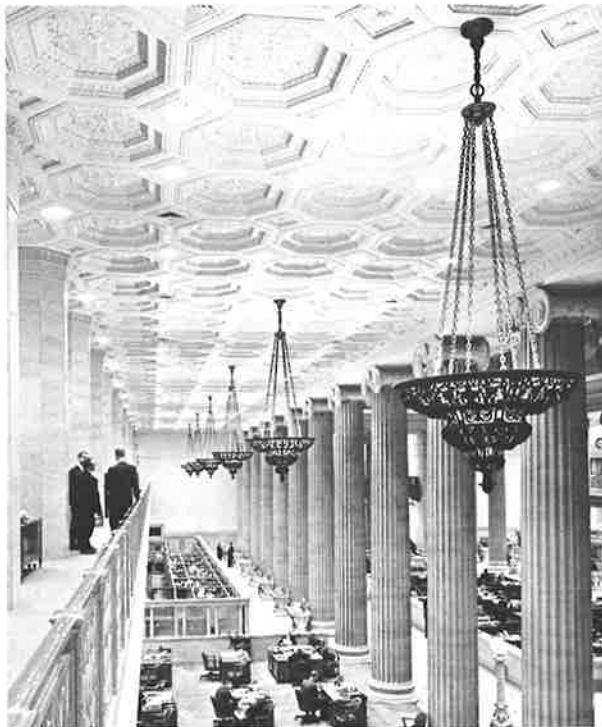
Decorative ceiling details are revealed when lighted. Here, lamps were mounted in the chandeliers and aimed toward the ceiling. Floor surfaces were sufficiently high in reflectance to "bounce" light back to the ceiling from the Quartzline lamps recessed in the smaller medallions in it.
