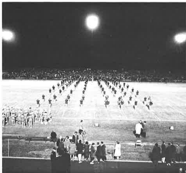
Quartzline lamps and fixtures provided good visibility for spectators, good color rendition, and low initial system costs. The narrow vertical beamspread and sharp cutoff characteristics of these units permits cross-aiming to the opposite side line. Wide horizontal beamspreads of fixtures meant that only six poles instead of eight were needed.
