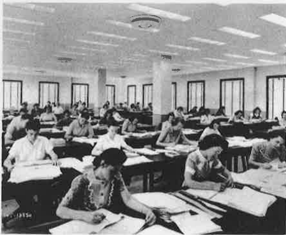
Fig. 4—Brightness-contrast, between lighting units and ceiling is low; glare is minimized. Work sheets happen to be large, thus surroundings of the task are bright and seeing conditions good.
