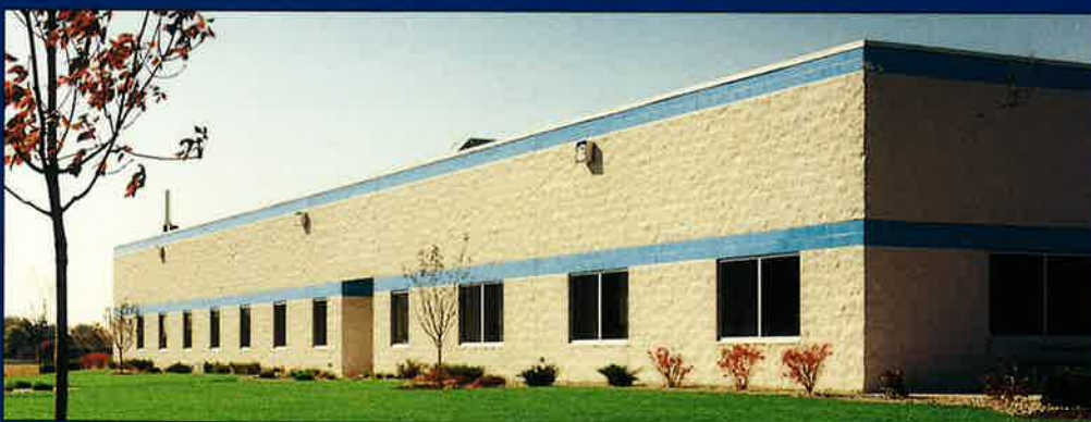
APL's 30,000 square foot facility is located on a 30 acre parcel of land in Urbana, Illinois.
