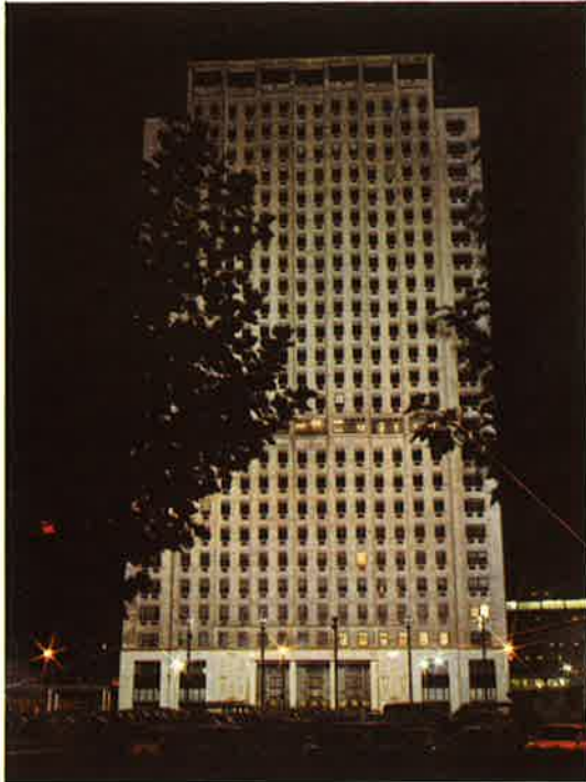
Left/ Prestige buildings come to life at night with Atlas discharge floodlighting.
