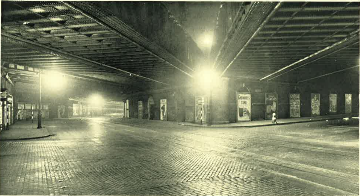
Railway Arches at King's Cross lighted by "Sieray" Lamps in Sussex-Sieray and Gower-Sieray Lanterns.
