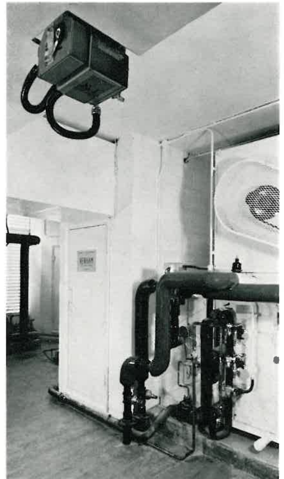
Part of the plant room
