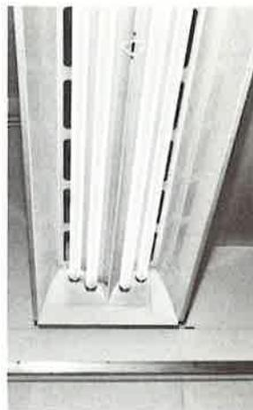
This fixture was designed at Nela Park, and is now available from several manufacturers. It has four high-output lamps, each eight feet long. There is an upward light component and 35° shielding. Light output is high — resulting in lower initial cost. Low operating costs result from the long life and good maintenance characteristics of the high-output lamps.
