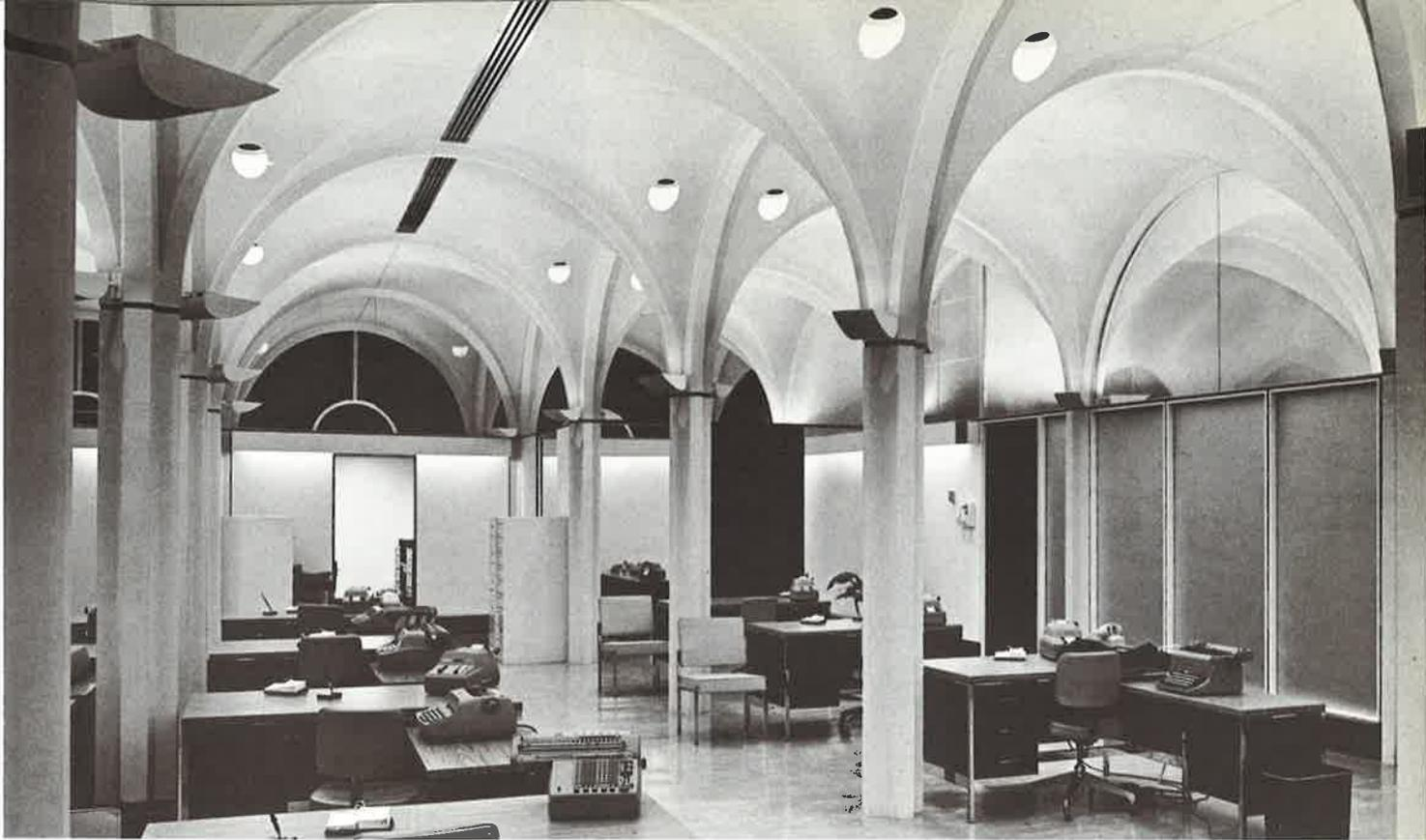
Vaulted ceilings, sweeping, soaring ceilings have, traditionally, been difficult to light effectively and efficiently. Now, compact, high-intensity sources may be placed in small units on columns, in coves, in recessed downlights . . . to produce light of coolness or warmth—wherever needed.
