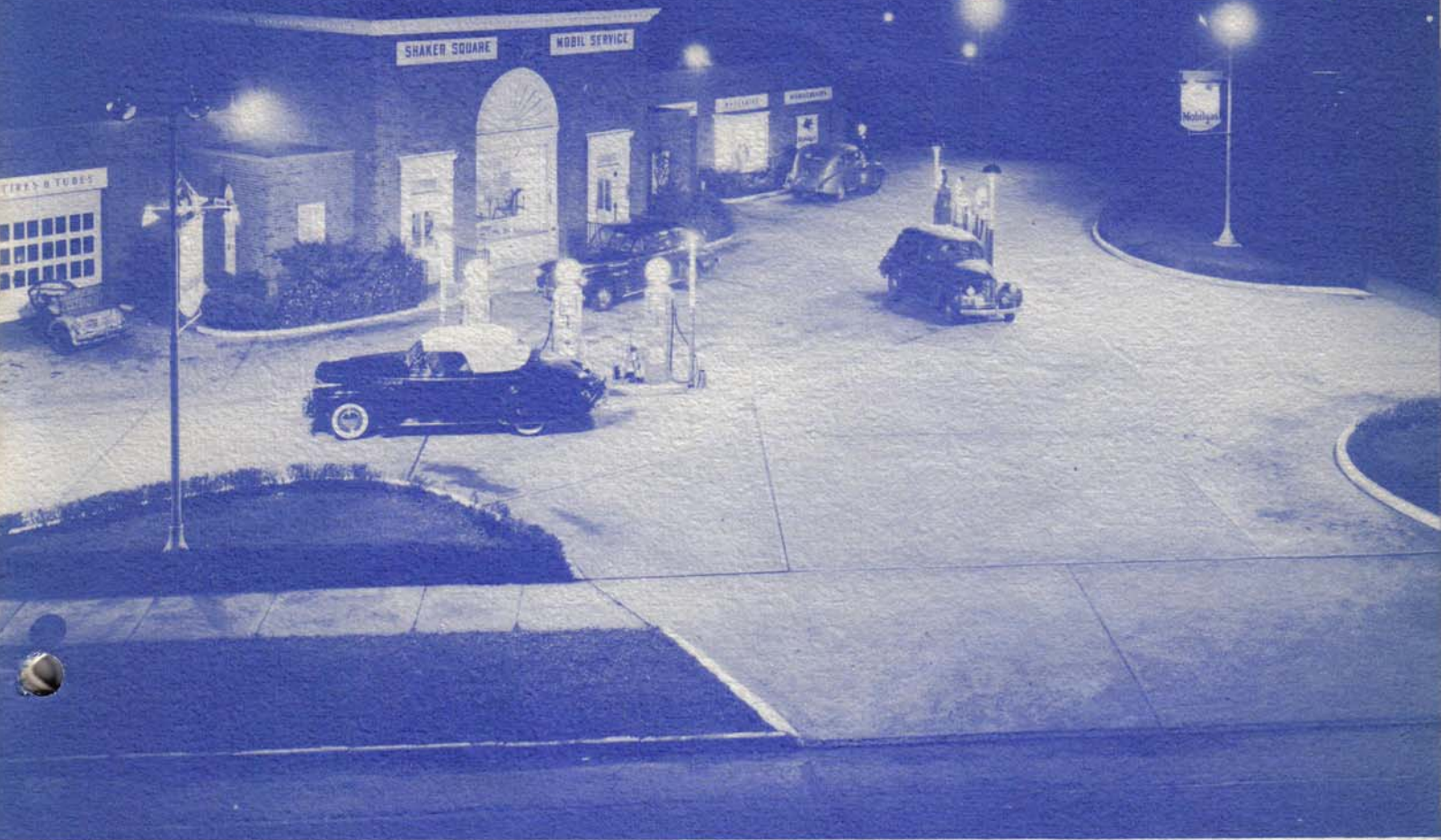
Attractive nighttime appearance of gasoline station provided by 400 watt A-HI or E-HI lamps in floodlight units. Warm color of light from incandescent lamps is used to light the pump island.
