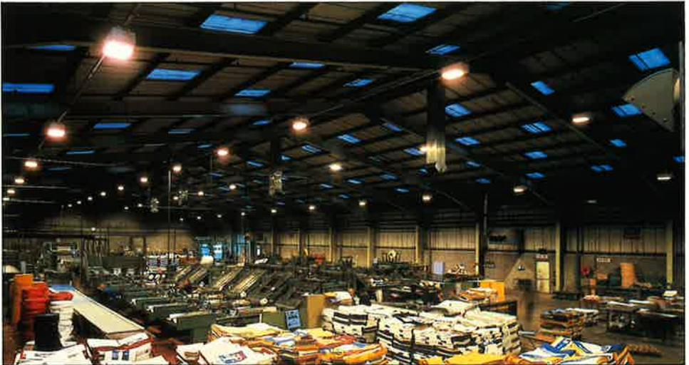
44 THORN EMI SON Deluxe lamps in Lopak fittings replaced 64 fluorescent fittings in Abertay's Paper Sack Company, cutting the previous electrical loading by nearly one third and increasing the illuminance level by one third.
