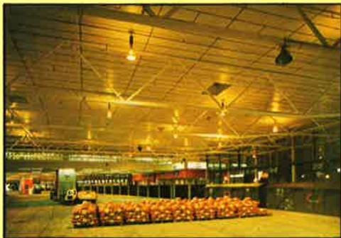
Transfesa Terminals Ltd. wanted pleasant working conditions and low running costs for their new ¼ mile long, covered rail head at Paddock Wood, Kent. Solarcolour (SON-R) reflector lamps provided the answer and over 300 are used to light the building which receives imported goods for onward distribution to all parts of the country.
